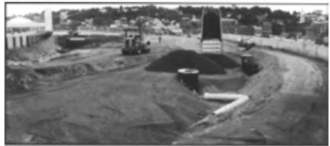
Retaining wall backfill, Providence, Rhode Island
